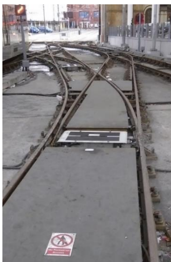
Figure Ap2.4: Infill Panels Shaped to Extend Through Points
