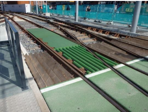
Figure Ap2.9: Application of Half Cylinder Panels (note that anti-pedestrian signage had not yet been fitted in this example)
