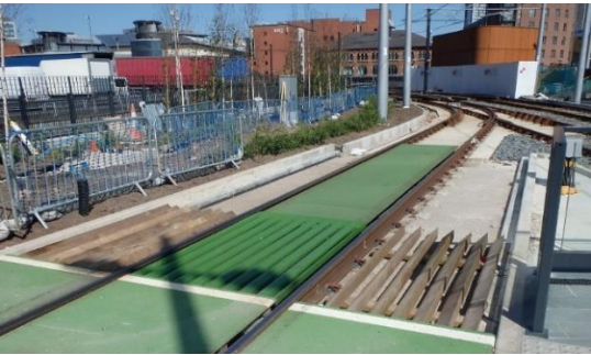
Figure Ap2.8: Application of Half Cylinder Panels (note that anti-pedestrian signage had not yet been fitted in this example)
