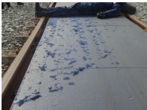
Figure Ap2.1: Standard Panels with Aggressive Non-slip Surface
