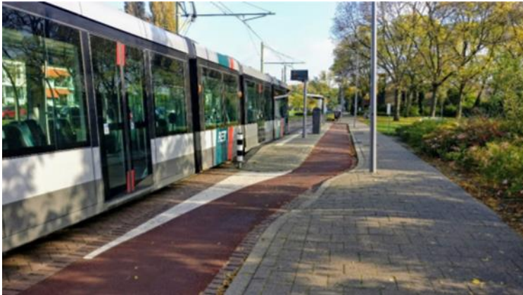
Figure 4.3 Cycle Bypass at Tramstop
