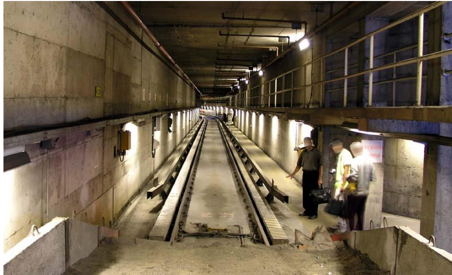
Figure 7: Sand Drag on Montreal Metro, similar to those on London Underground but deeper across the full width of the track
