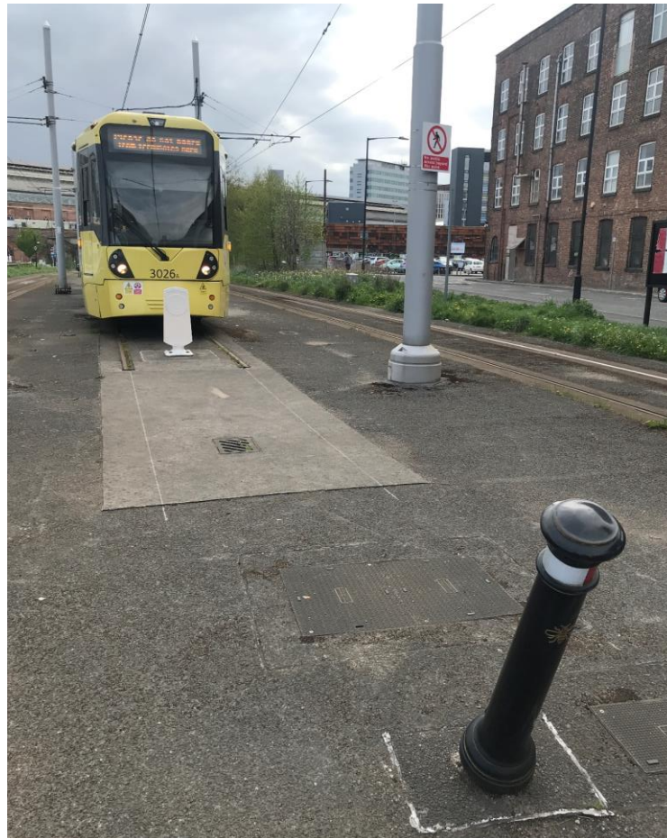
Figure 16: ‘Two nice parallel lines and a wonky bollard’ [19] Evidence of the Sheffield Street over-run: the flush surfaced arrestor bed (grey rectangle) did not function as intended.
