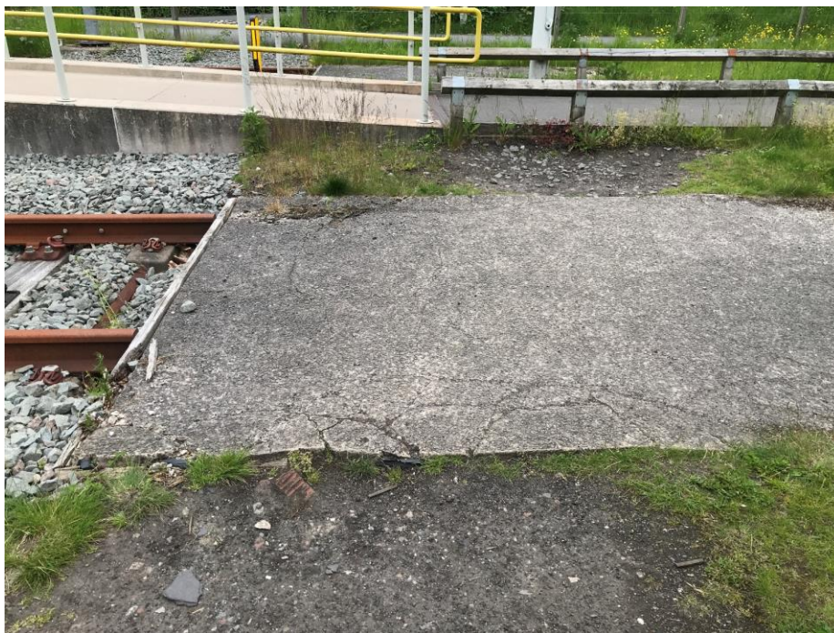
Figure 18: Flush surfaced arrestor bed at East Didsbury, breaking up under pedestrian traffic
