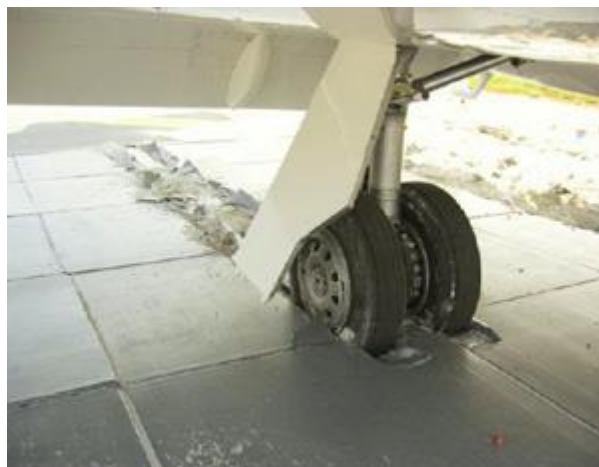
Figure 22: EMAS system showing the blocks crushed locally under the aircraft wheels [31]
